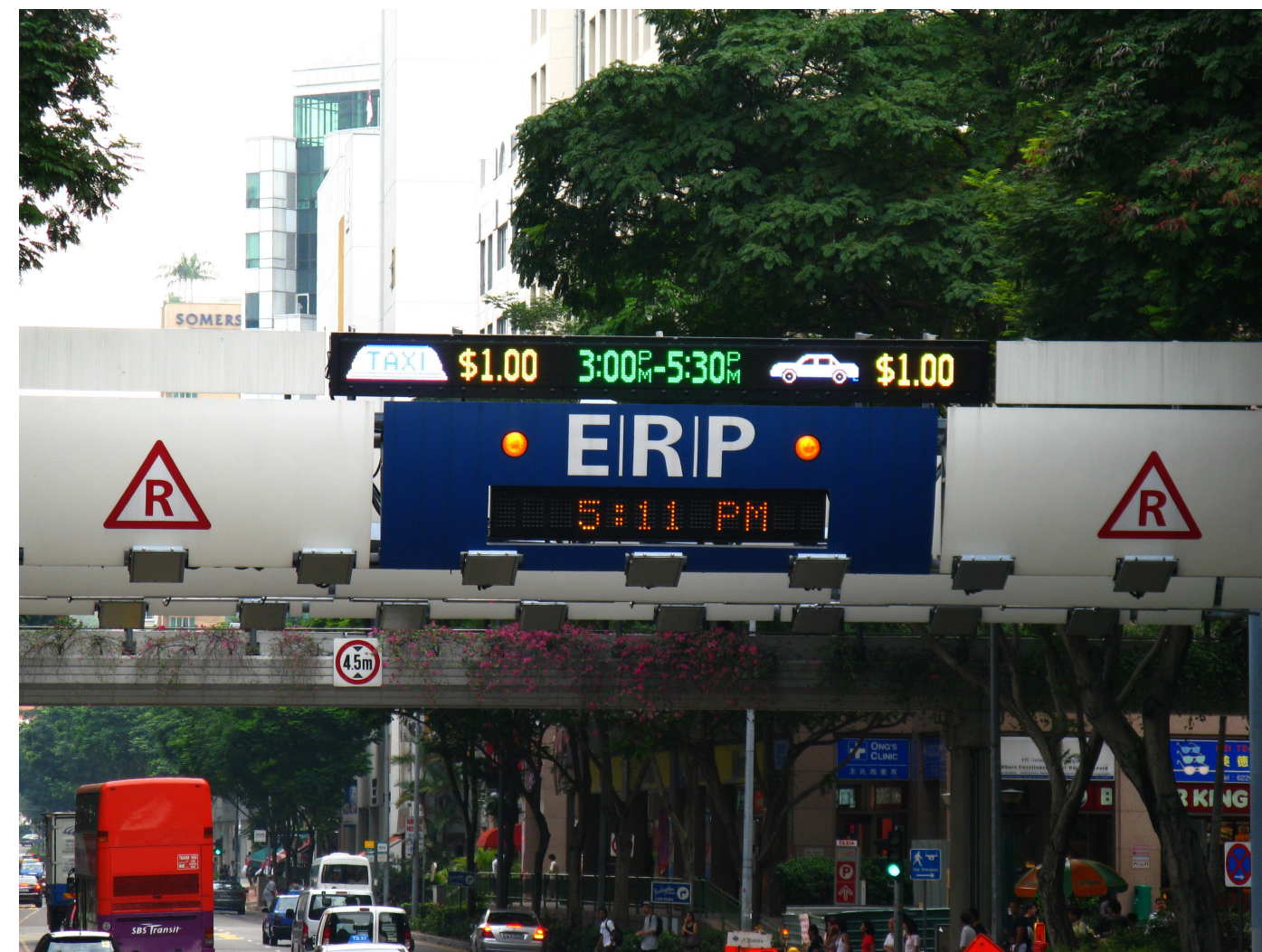
An electronic toll gantry equip with cameras that can read license plates
