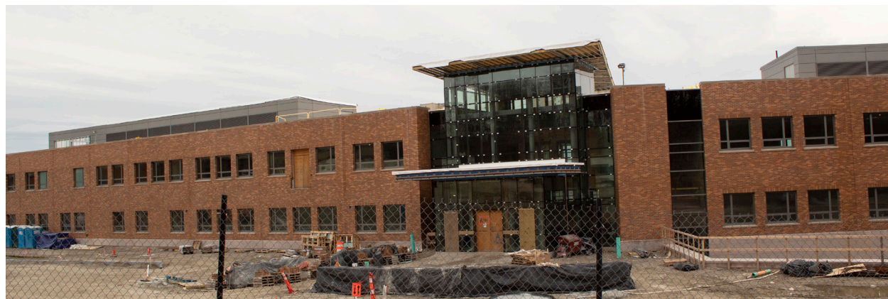
The new Grasso Tech building in progress
