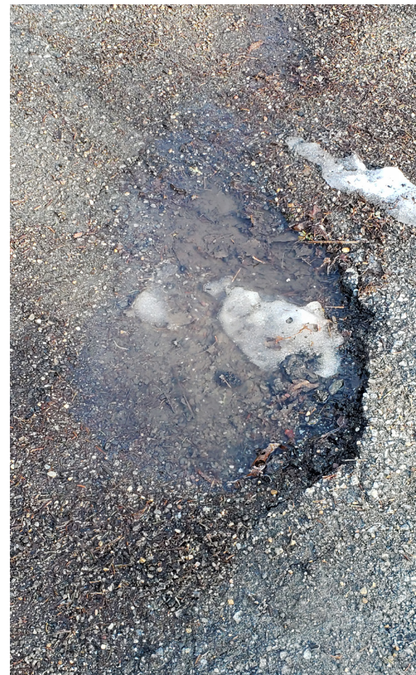
Pothole courtesy of Hope Whiteley
