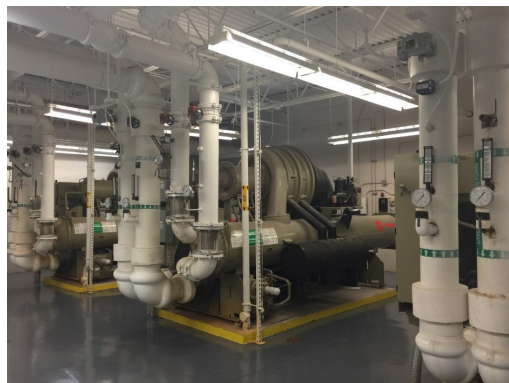
FIGURE 2.3: Centrifugal Water Cooled Chillers
