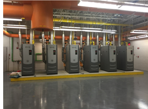
FIGURE 2.4: Cascaded Benchmark Condensing Boilers
