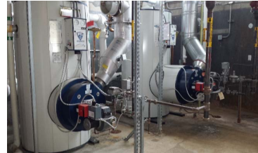
Domestic Gas Fired Hot Water Heaters
