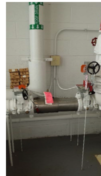
Fire Service Backflow Preventer
