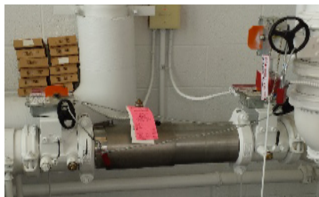
Fire Service Backflow Preventer
