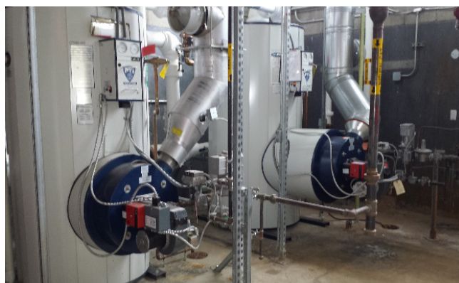
Domestic Gas Fired Hot Water Heaters
